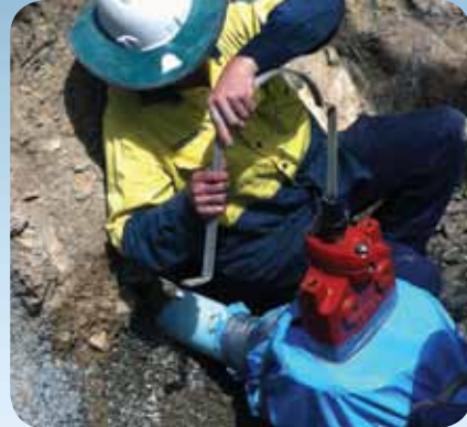
An InsertValve installation under full line pressure.
